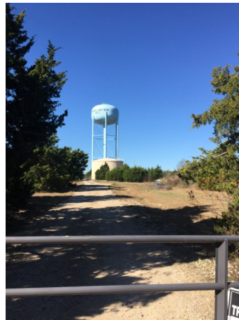
Sardis-Lone Elm Water Supply is one of the recent additions in the district monitor well program.
