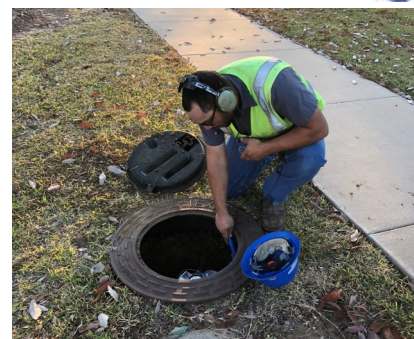
Another utility employee uses acoustical leak detection equipment on a water valve.
