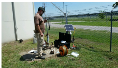
Equipping a new monitor well in Aquilla
