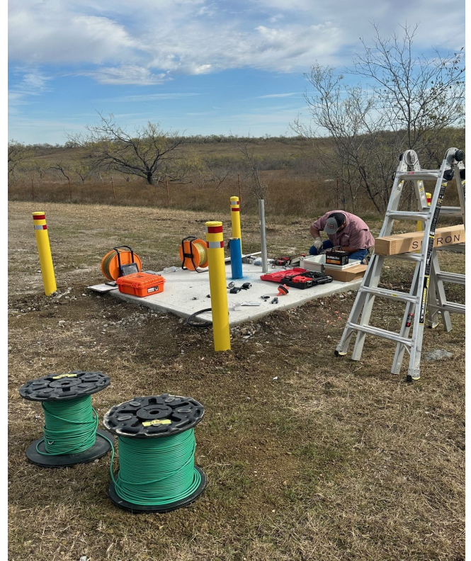
Field Technician, Jose Sarmiento, installs equipment on newly drilled monitor well.
