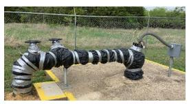
components. Begin by insulating exposed pipes and components to prevent freezing. Cleaning out enclosures provides room to insulate above-ground water lines and other components, such as pressure tanks. Ensure that all vital above-ground components are protected with insulating material, and wrap plumbing from the well to storage tanks with insulation to prevent freezing. The smaller the pipe in diameter and closer to the ground, the more vulnerable it is to freezing.
