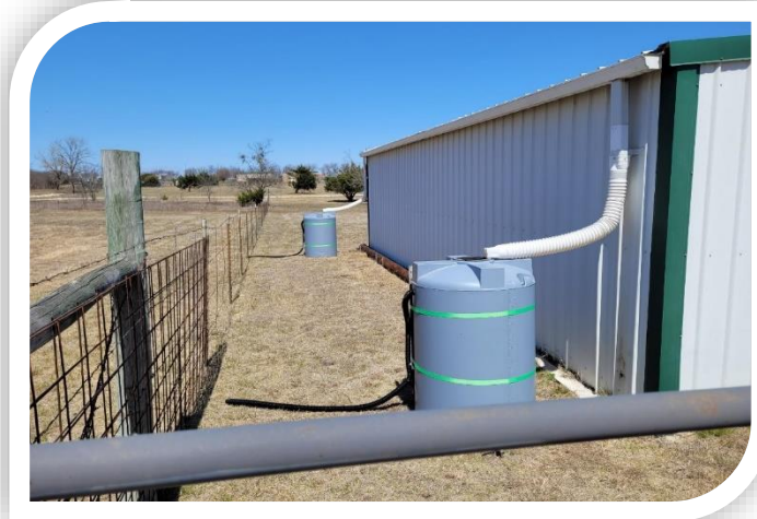
Private Residence, Johnson County
