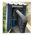
Please take this opportunity to inspect your well casing and the ground around it. Ensuring that there are no holes in or around your well casing, including at the ground level, so that burrowing critters have no pathway to contaminate your well. By adding dirt or concrete around your well, you are protecting them from rain and other runoff water and making sure there is a pathway for it to move away from your well and not pool up around it.
