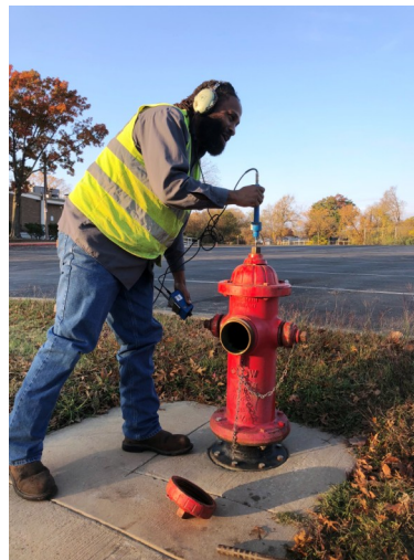
A water supply employee listens for leaks on a water main via a fire hydrant.
