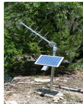
Monitor equipment is solar-powered and data is transmitted via satellite uplink.
