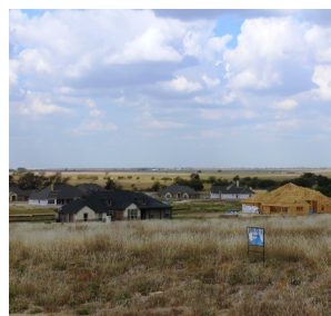
Johnson County subdivision with numerous new homes—all with a residential well screened at the same level in the same aquifer.
