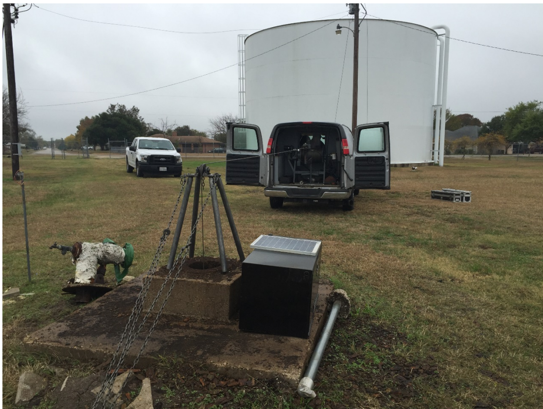
Pulling a pump to install monitor equipment
