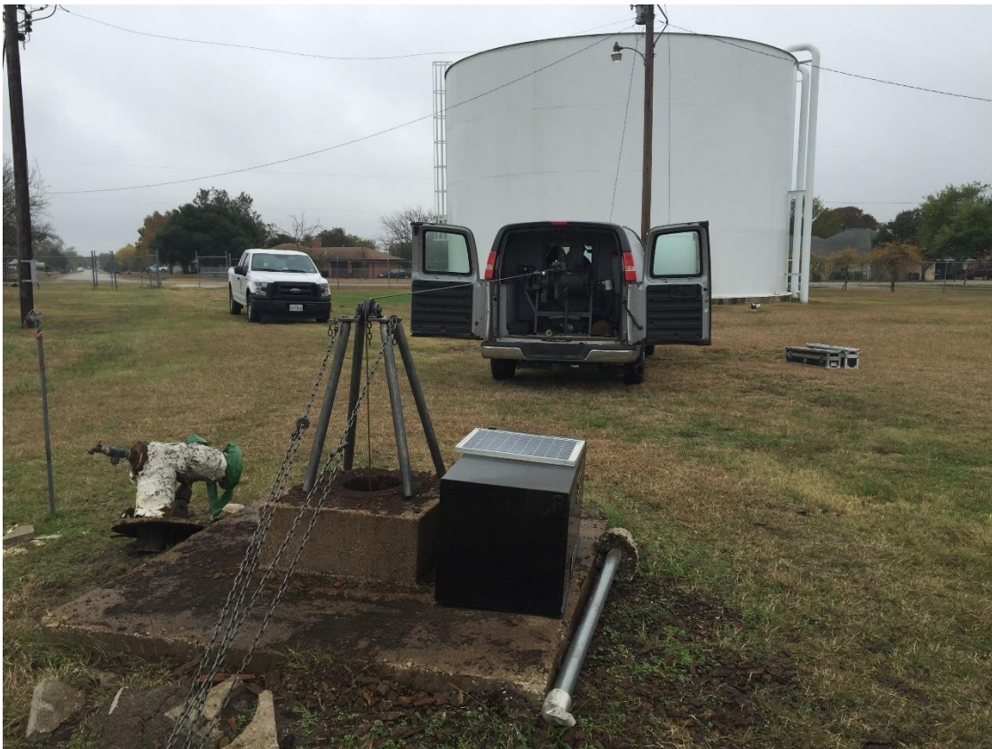
Pulling a pump to install monitor equipment
